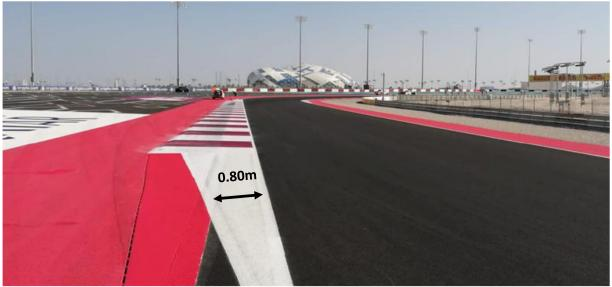
The track edge between Turn 13 and Turn 14 on LHS has been moved by approximately 0.80m to the right.
